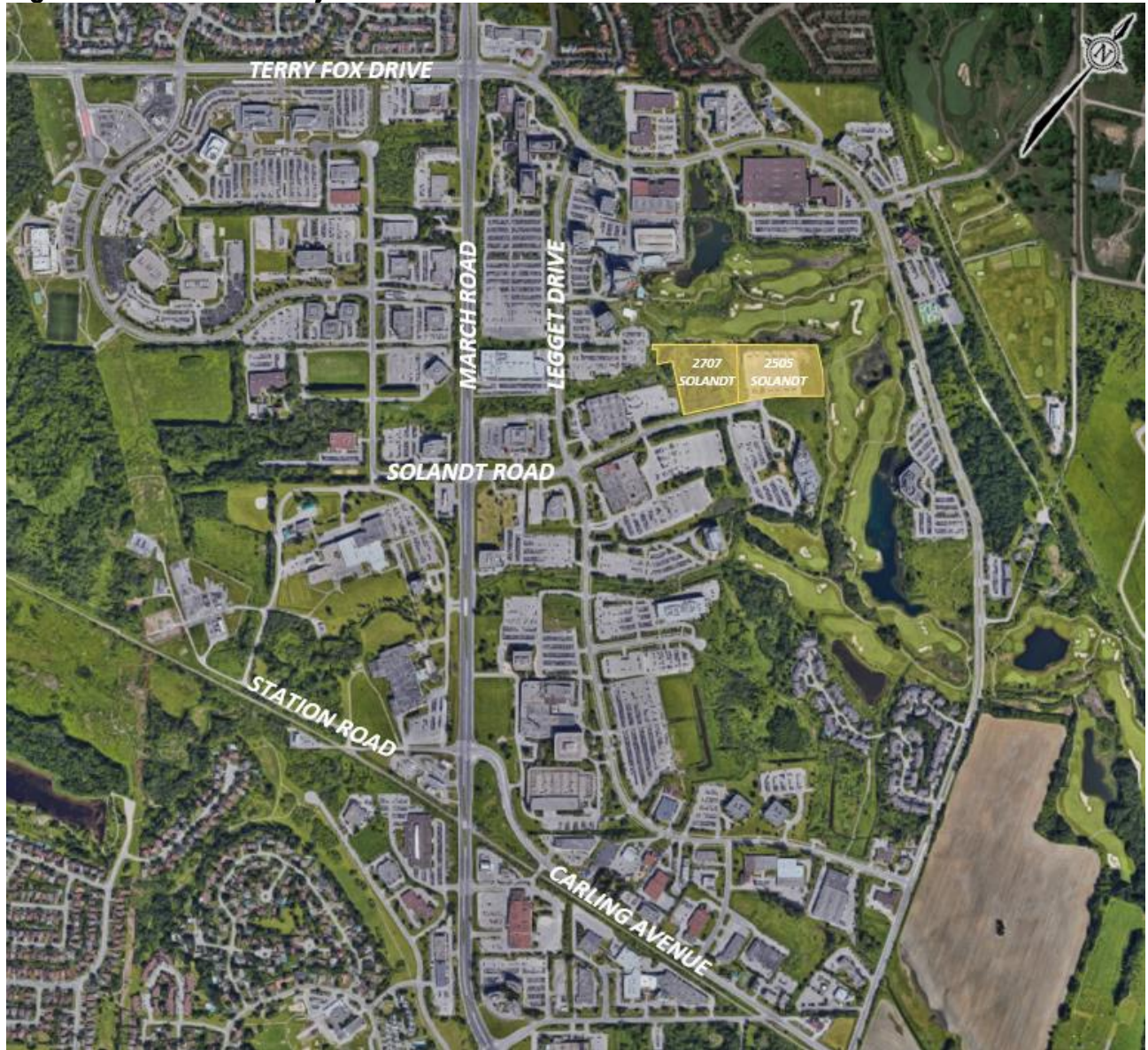
Figure 1: View of the Subject Site
