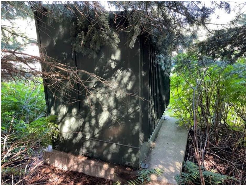
**Photo 14:** 2001 manufactured pad mounted, oil filled transformer along northern property boundary.
