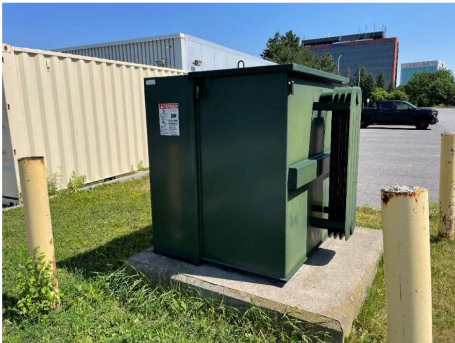
**Photo 16:** Transformer supplying power to the 555 March Road building. Unknown filling.
