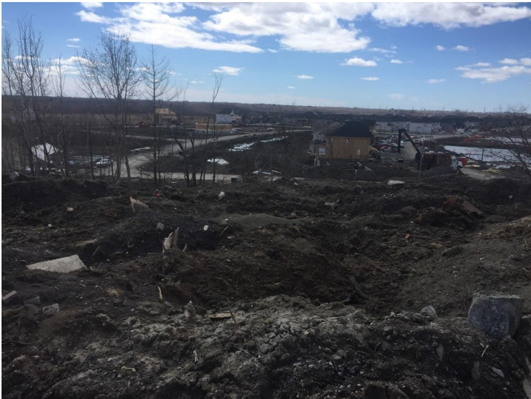
Photograph 4: Central portion of the site, facing west
