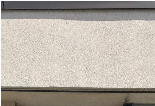
Figure 23. Aggregate-faced concrete paneling (ERA, 2021).
