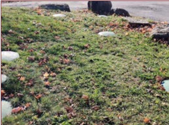
Photograph I11 – One of the several septic systems located on the Site.
