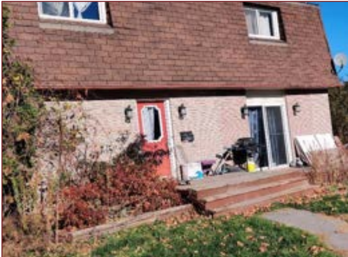
Photograph I15 – One of the structures (1090 Antochi Lane) located at the Site.
