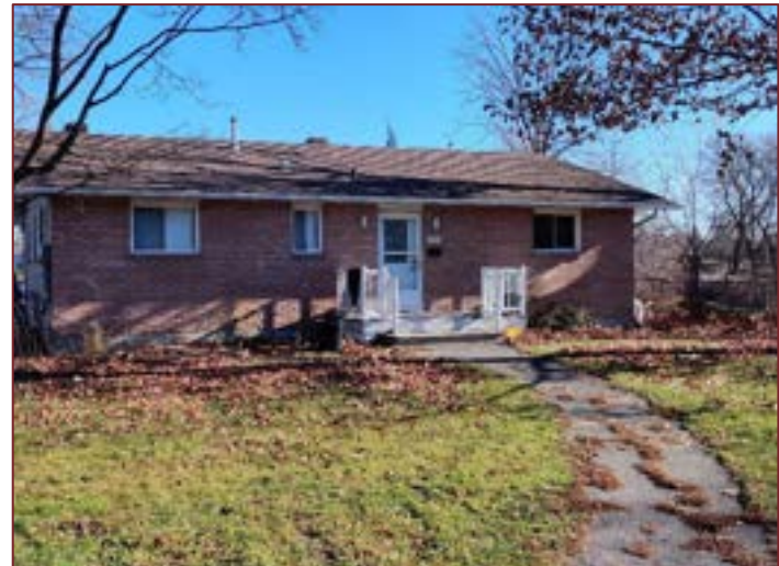
Photograph I16 – One of the structures (1087 Antochi Lane) located at the Site.
