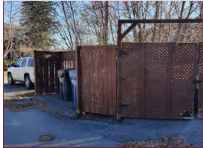
Photograph I10 – Garbage disposal area (located centrally) and is managed by a contractor on a weekly basis.
