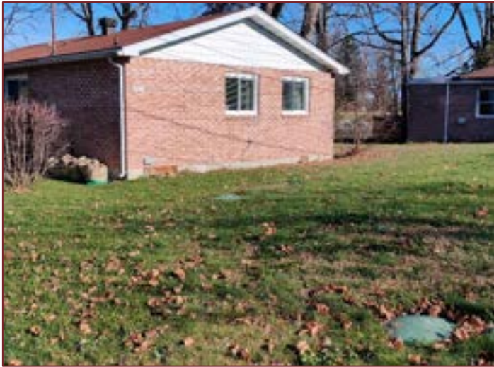
Photograph I13 – One of the structures (1097 Antochi Lane) located at the Site.
