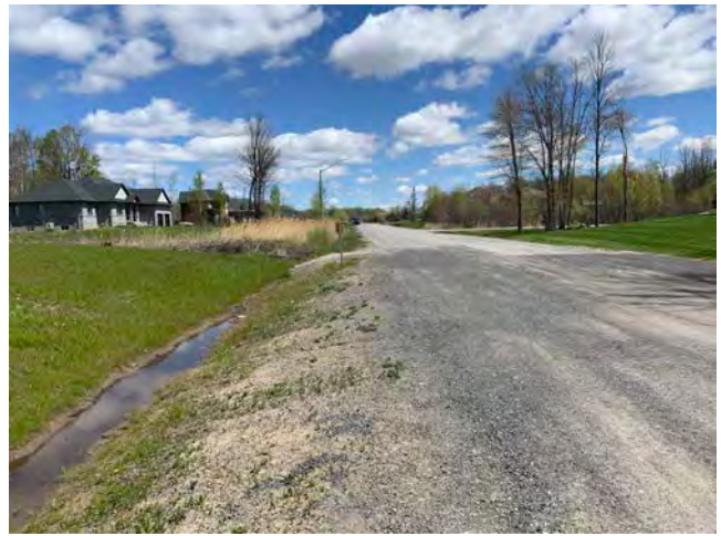
Photo 2: Existing conditions observed within the existing Emerald Creek subdivision along Tullamore Street immediately east of the Site (May 6).
