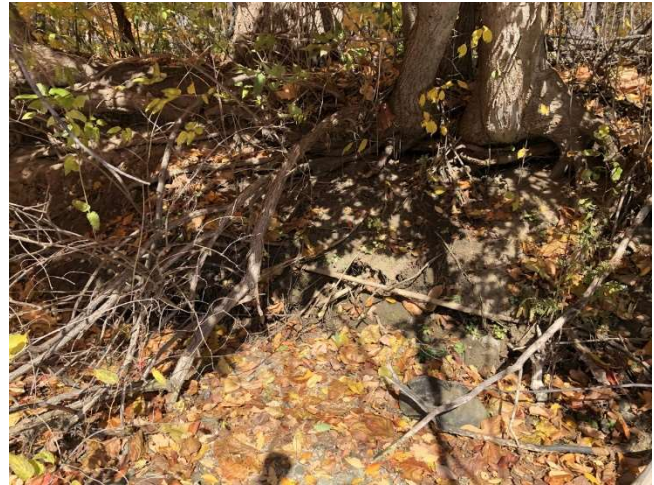
Photo 2: View looking at S2 (perpendicular to bank) on October 14, 2022.
