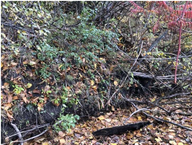
Photo 21: View looking at S21 (perpendicular to bank) on October 14, 2022.
