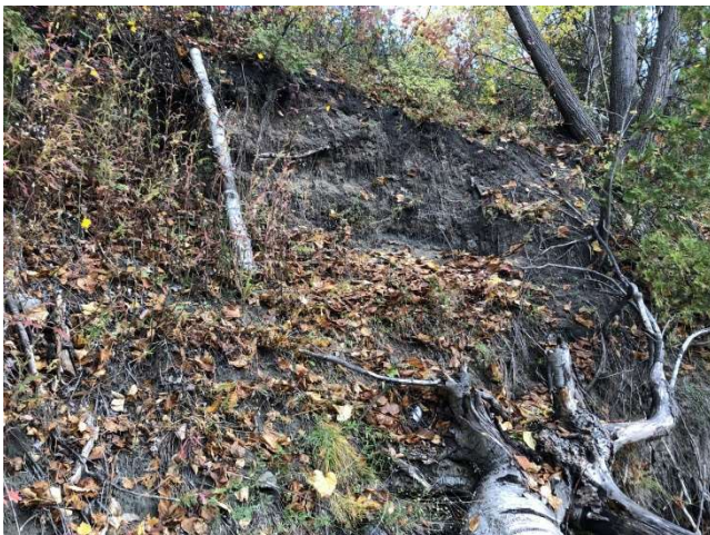
Photo 17: View looking at S17 (perpendicular to bank) on October 14, 2022.
