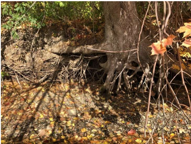
Photo 9: View looking at S9 (perpendicular to bank) on October 14, 2022.
