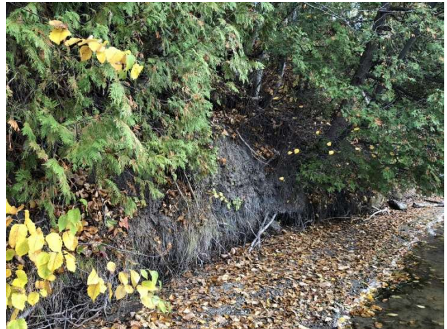
Photo 16: View looking upstream at S16 on October 14, 2022
