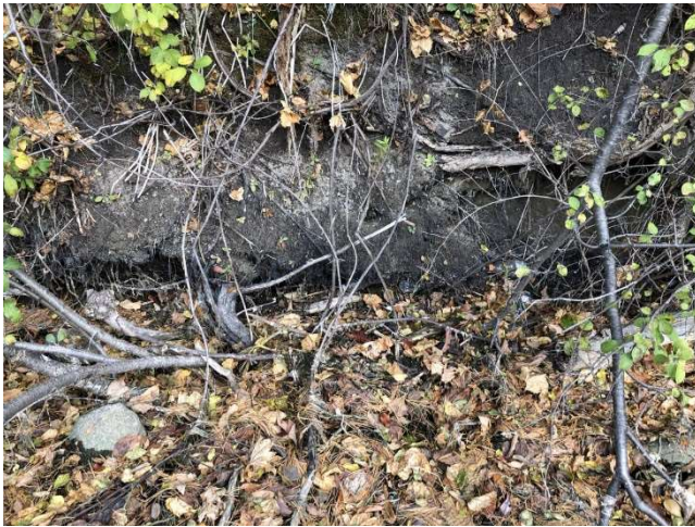
Photo 13: View looking at S13 (perpendicular to bank) on October 14, 2022.
