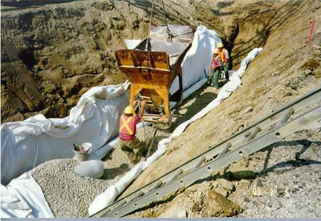
Figure 12 Backfilling of perforated pipes
