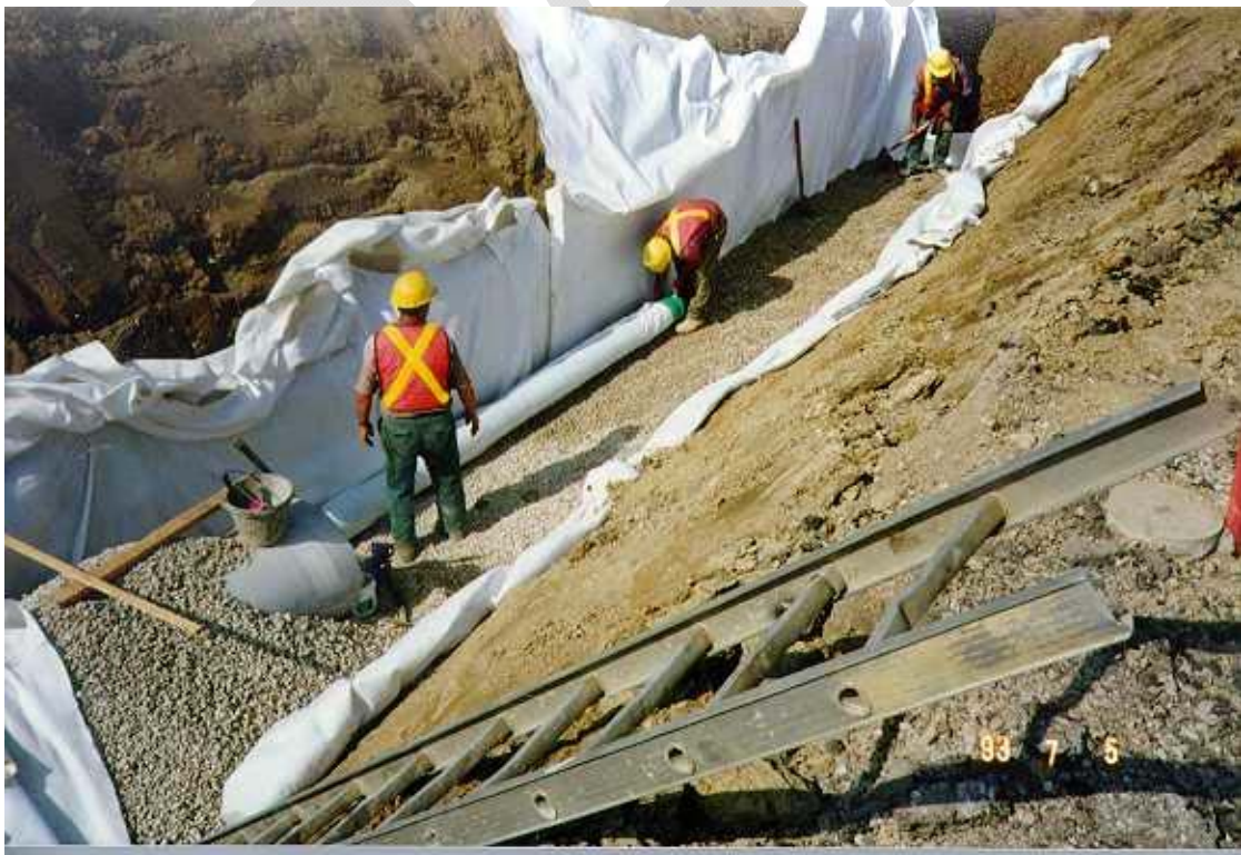
Figure 11 Laying of perforated pipe at sewer trench
