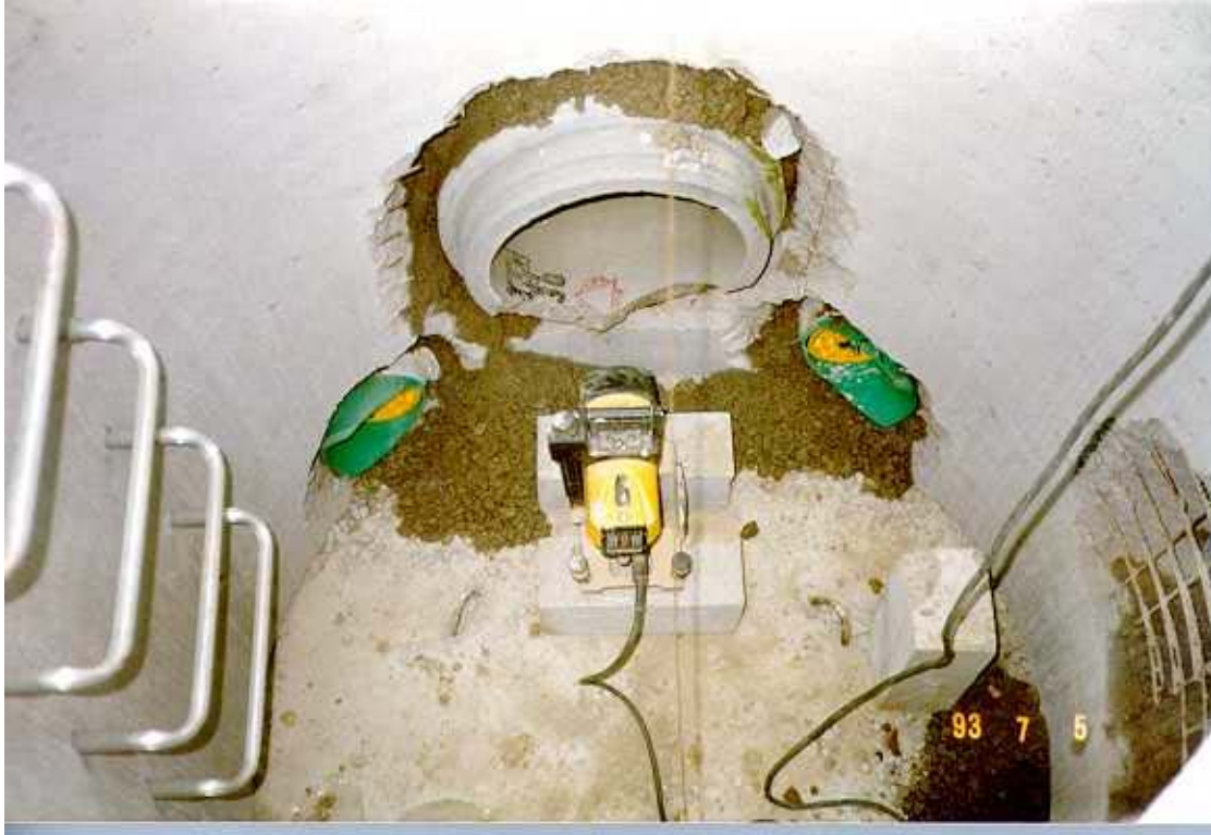
Figure 16 Mechanical plugs installed at the downstream end of perforated pipes
