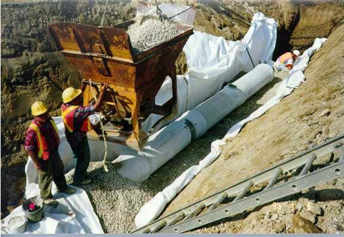
Figure 14 Backfilling of storm sewers
