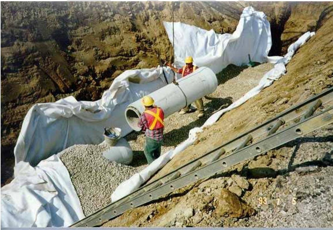
Figure 13 Laying of storm sewers on top of perforated pipes
