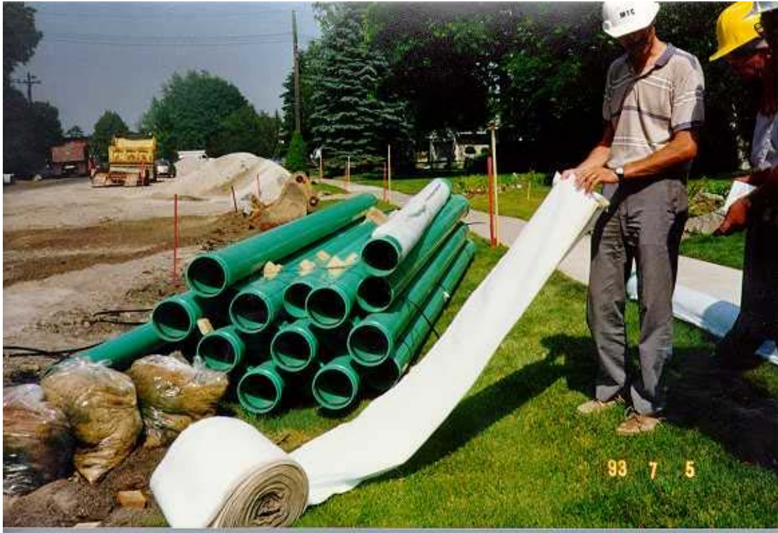
Figure 10 200 mm perforated pipes with filter cloth socks.
