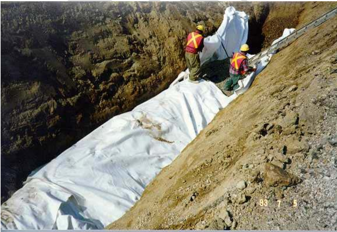
Figure 15 Wrapping of filter cloth around the stone trench
