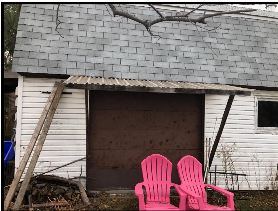
Photograph 6: Northern façade of two storey wood framed workshop, facing south.
