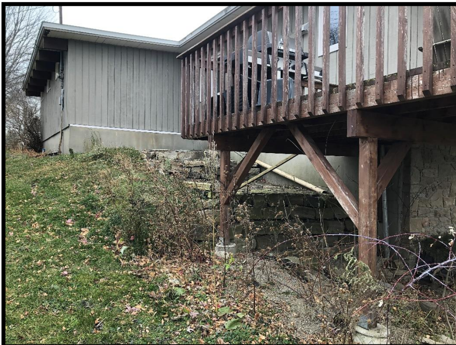
Photograph 4: Northern façade of residential dwelling, facing east.
