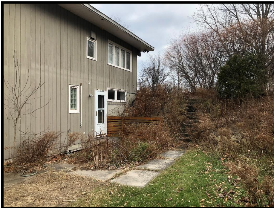
Photograph 2: Southern façade and side basement entrance of residential dwelling, facing northeast.
