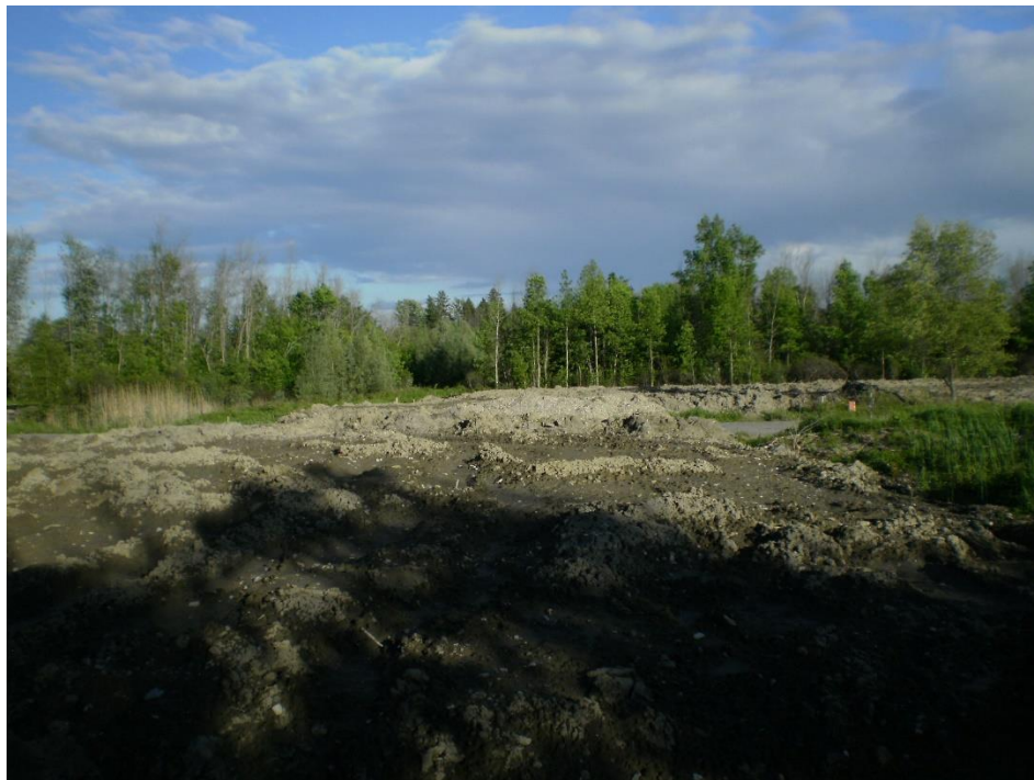
Photo 2 – Fill in the northwest portion of the Phase 3 lands, with view looking south to the Tullamore Street extension
