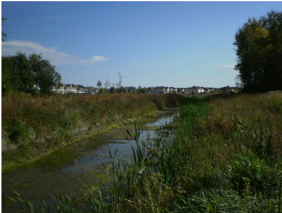
Photo 1 – Recently constructed north-south swale immediately to the east of the site. View looking south.
