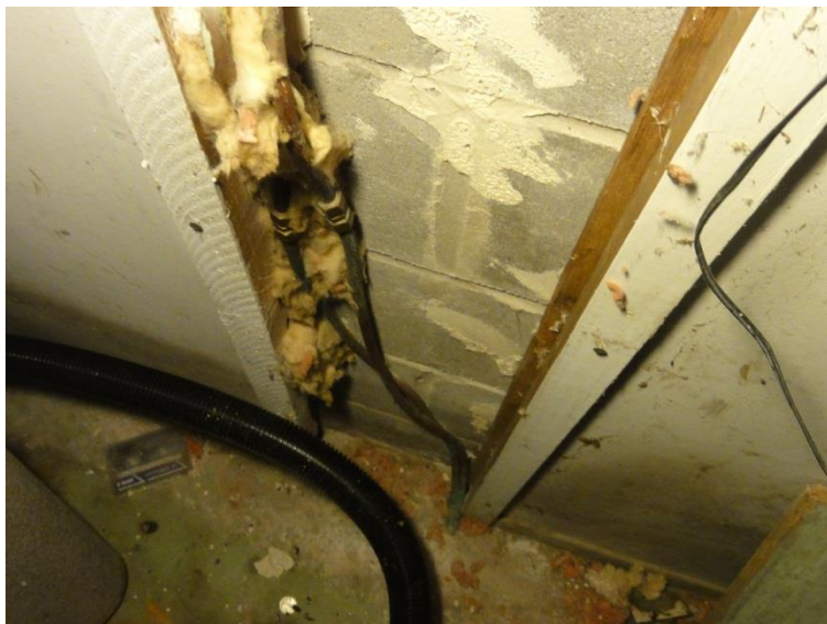
Photo 4 – View of potential UST feeder line observed in the basement furnace room of the residence, located along the inside wall adjacent to exterior vent/fill pipes.
