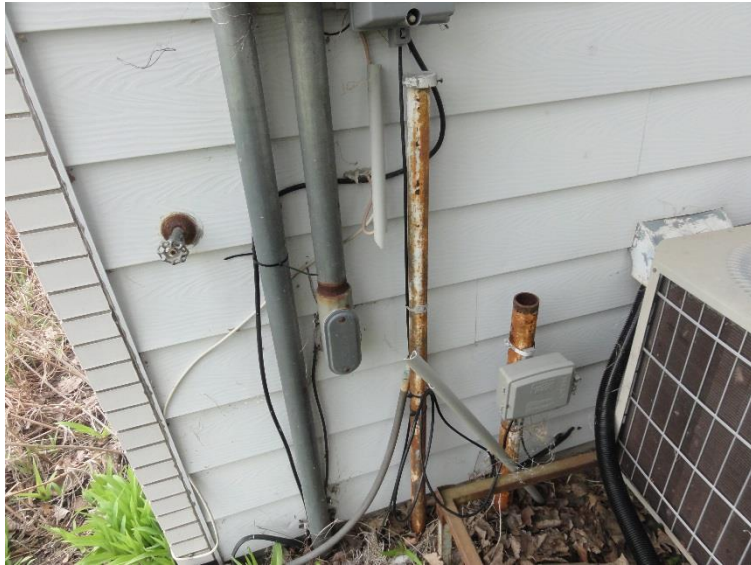
Photo 3 – View of vent and fill pipes, likely associated with former UST, entering the ground on the northeast corner of the residential building.
