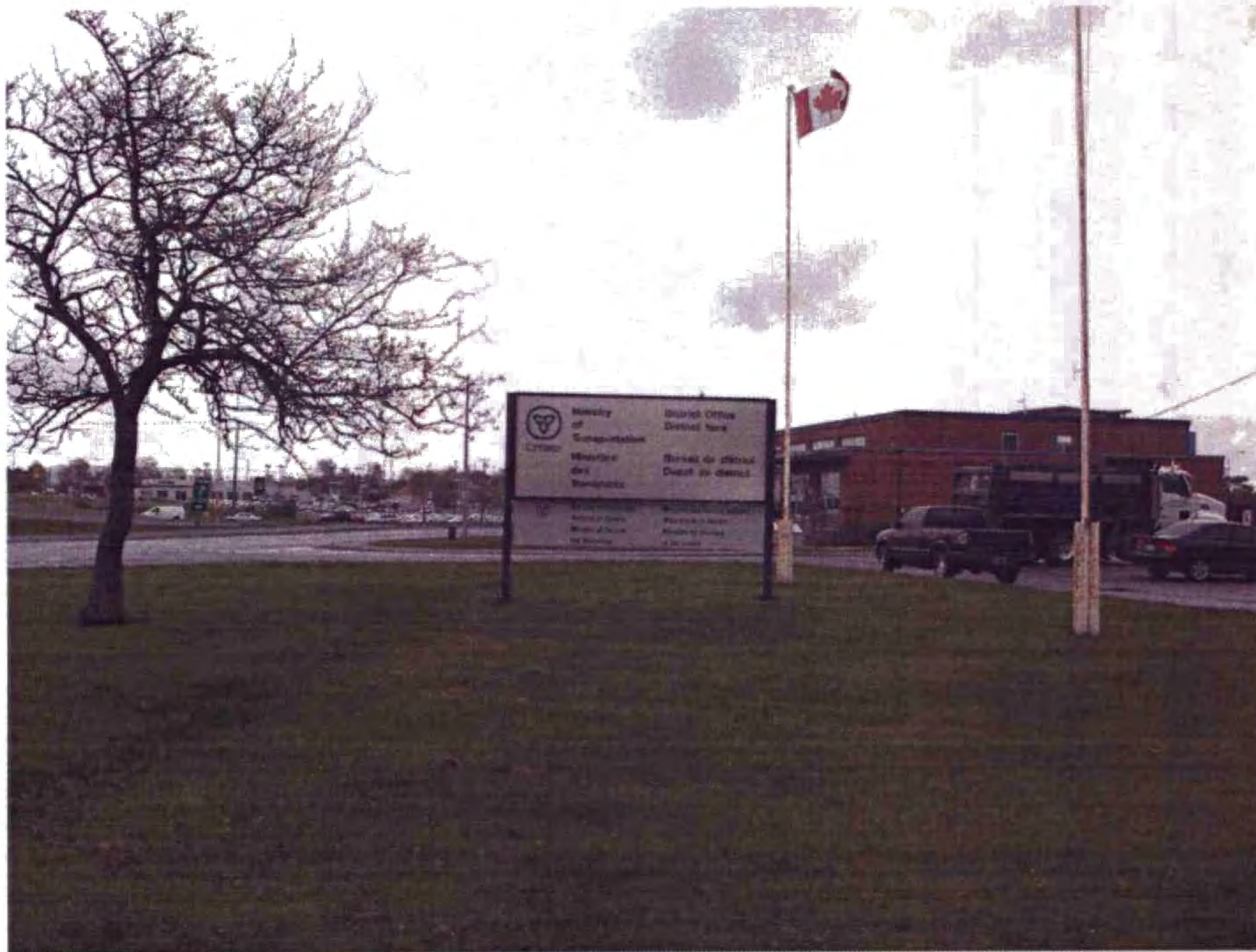
Figure 3: MTO Facility Fronting Tremblay Road, looking east
