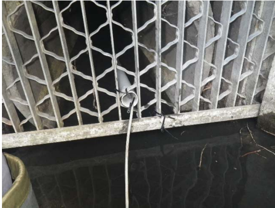
Figure 2a: Stingray and water level logger Installation on culvert grate at Q1
