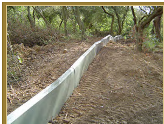
Plate 7. Pre-formed vinyl sheeting fence intended to exclude salamanders for a construction site (photo credit: Herpetosure Ltd.)
