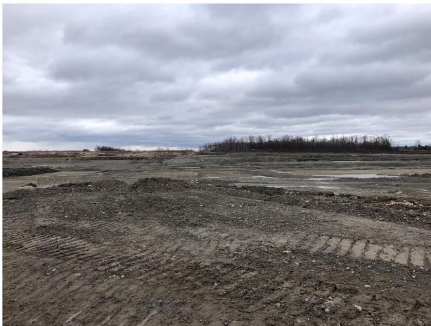
**Photo B3.** Southward view across the east end of the Brazeau site. The small slopes along the southern lot line are new features temporarily created as material is moved around the site. The slopes there are being maintained at a low angle and will disappear as fill is added to the foreground.
