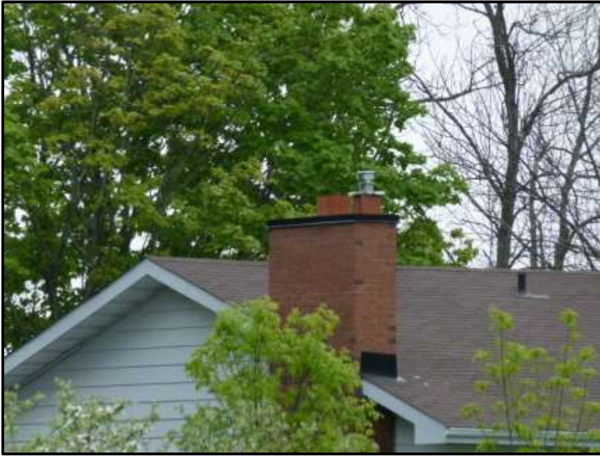
Photograph 35: Chimney at 1145 March Road. Note the ceramic liner and metal cap (May 24 th , 2017).
