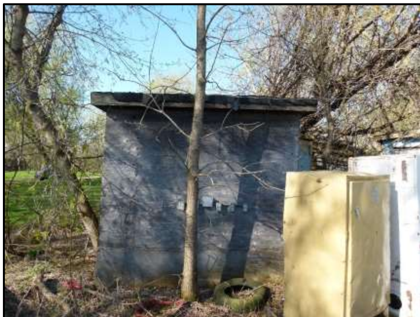
Photograph 43: Building #2 – Looking west at the small wooden shed (May 8 th , 2018).
