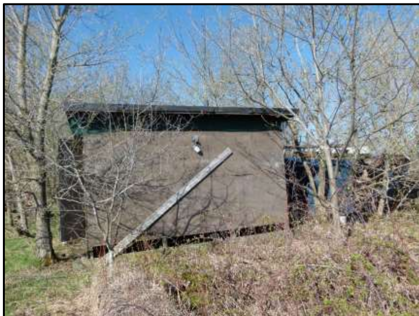
Photograph 44: Building #3 – Looking west at the medium wooden shed (May 8 th , 2018).
