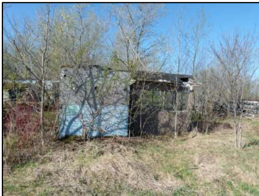
Photograph 45: Building #4 – Looking west at the small wooden shed and glass gazebo (May 8 th , 2018).
