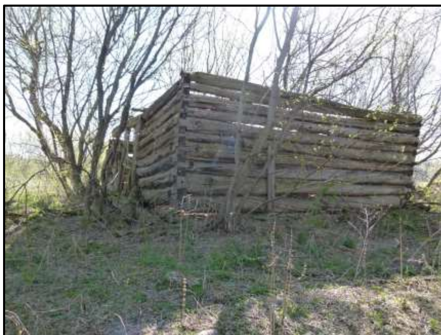
Photograph 46: Building #5 – Looking south at the old barn foundation (May 8 th , 2018).
