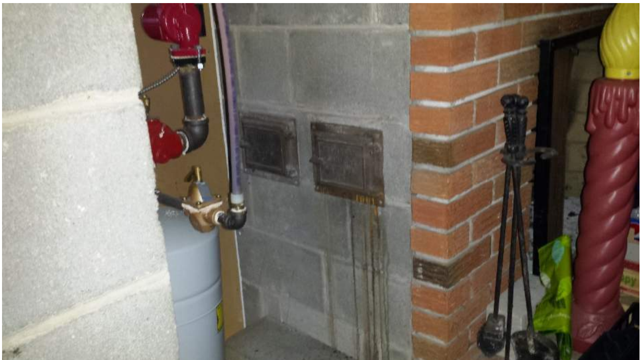
Photograph 8: Fireplace and cleanouts in the basement of 33 Deerfox Drive.
