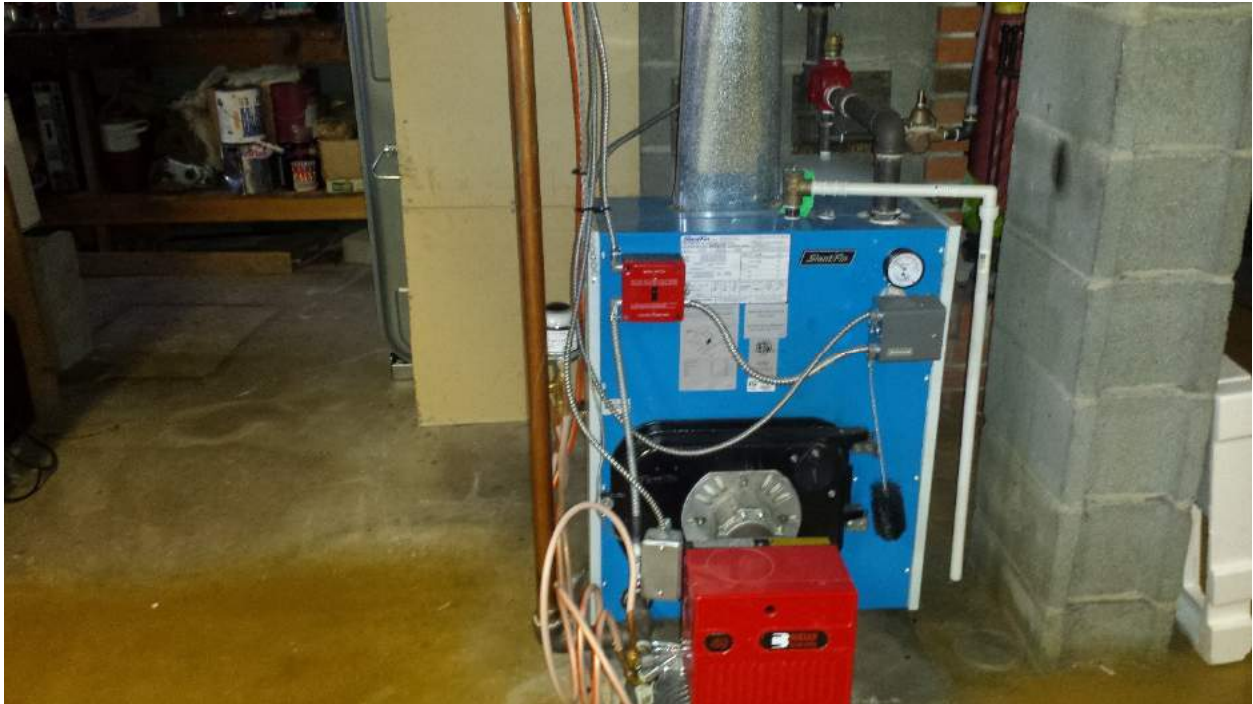
Photograph 7: Boiler in the basement at 33 Deerfox Drive, with the oil tank visible behind.
