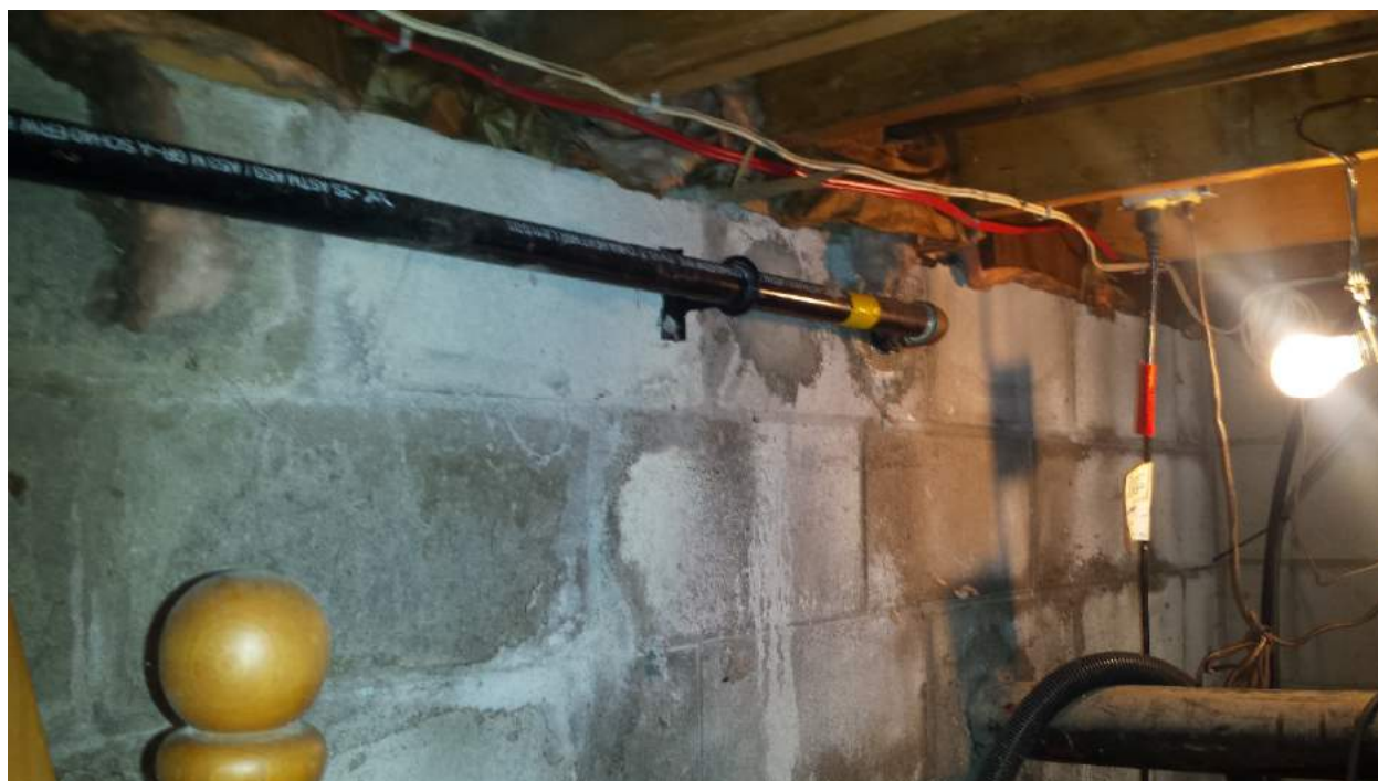
Photograph 3: The former location of a fuel oil tank at 23 Deerfox Drive. The vent and fill pipe holes have been patched in the concrete wall.
