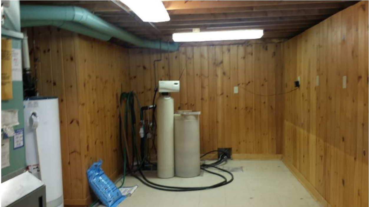
Photograph 9: Sump pit (left) and water softener in the basement of 39 Deerfox Drive.
