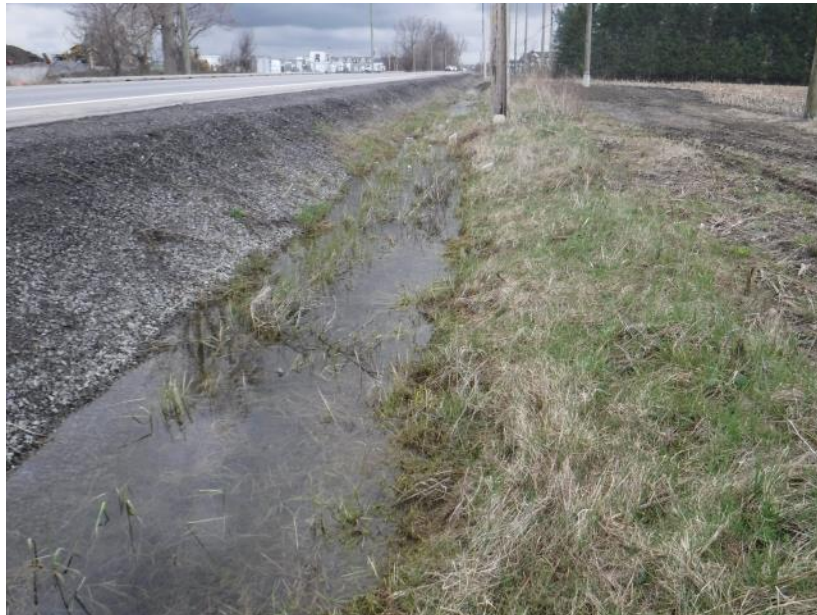
Photo 7 Station 3 looking upstream from the downstream end (May 2, 2016)
