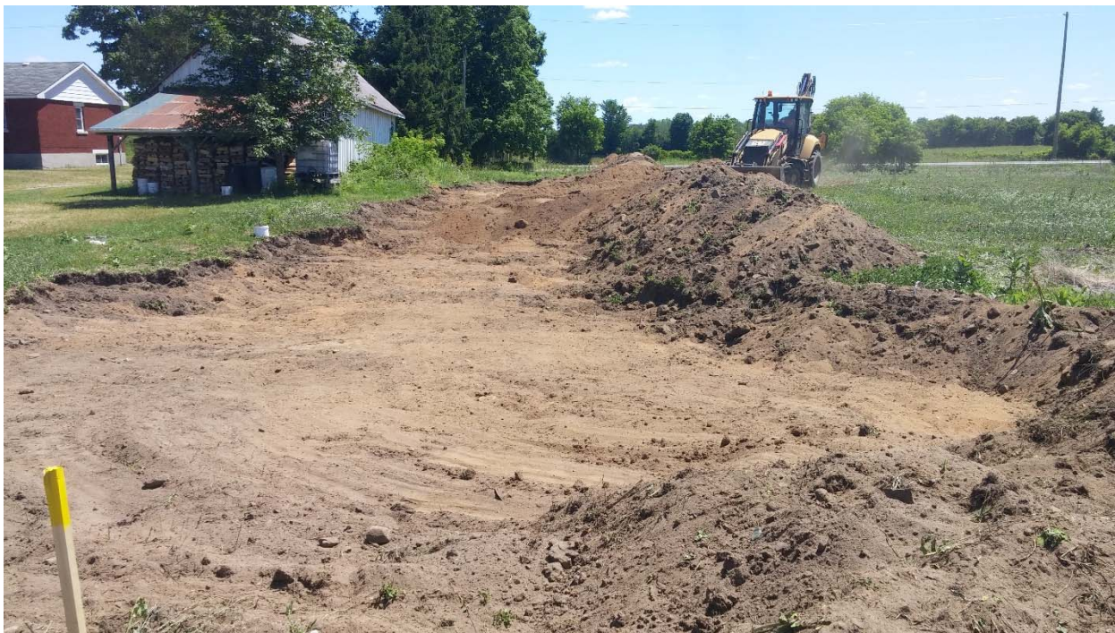
Image 8: Backfilling in eastern half facing southeast.
