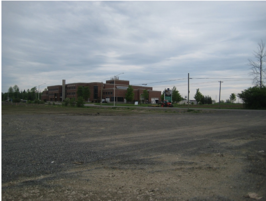
Photograph 1: View of the Site entrance from Greenbank Road looking north.
