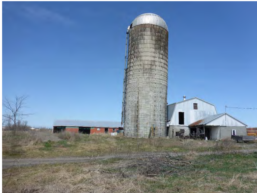
Image 4: Barn and outbuildings located in Operation 1, looking north (Photo Location 8).
