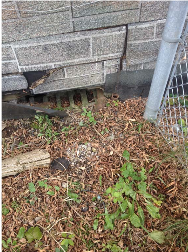
Fill Pipes for Above Ground Furnace Oil Tank located in basement of abandoned single family dwelling
