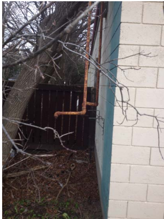
Disconnected Gas located at northwest corner of building (shop)
