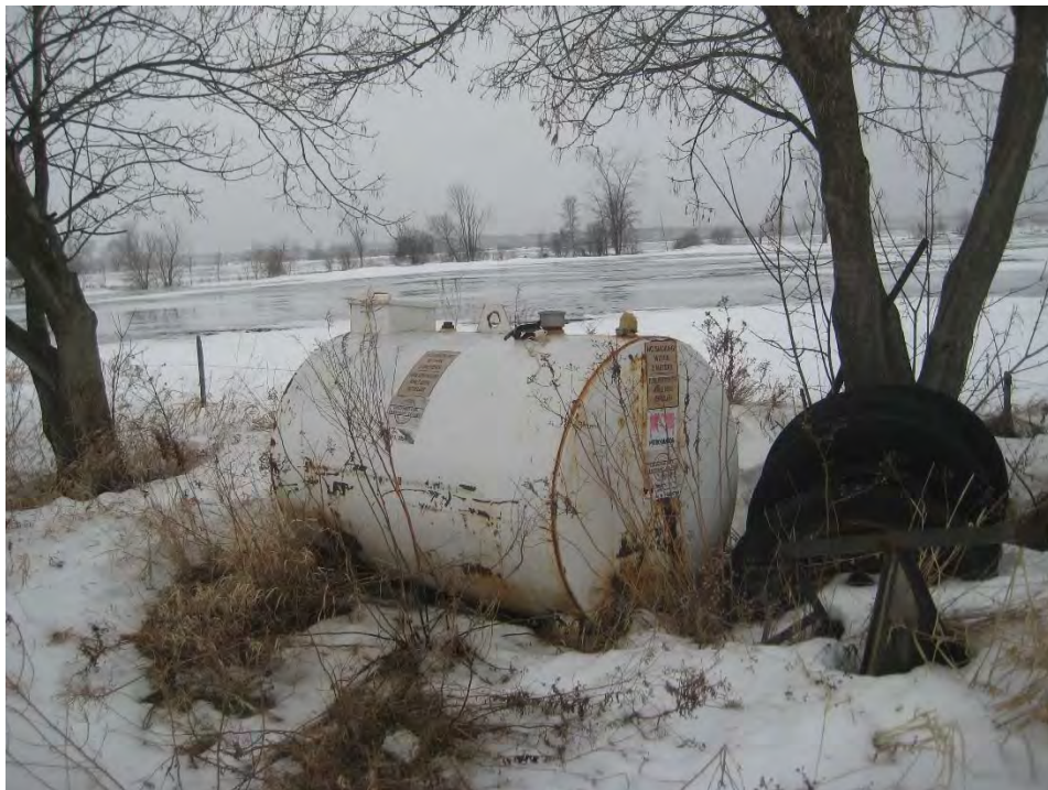
Photograph 24: View of the old discarded AST noted in the south part of the Site.
