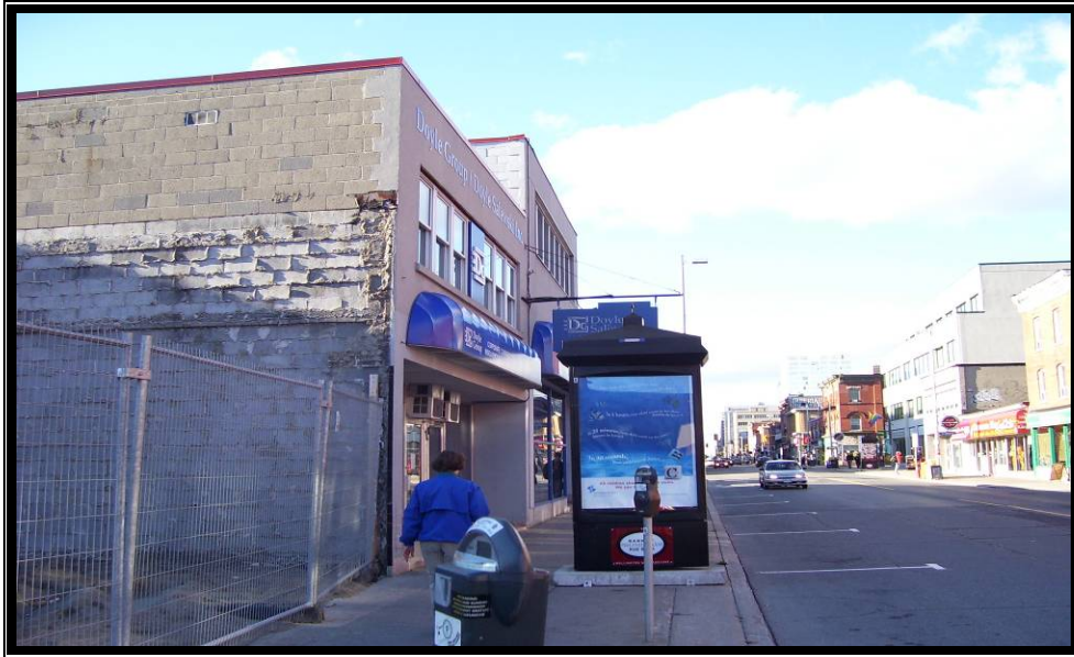
Photograph 3 – Adjacent properties located north of the Site.
