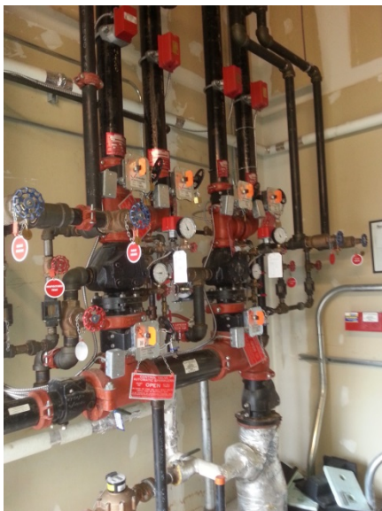
Photo 11 – Sprinkler system in the utility room in the commercial retail units. Insulation is fibreglass.
