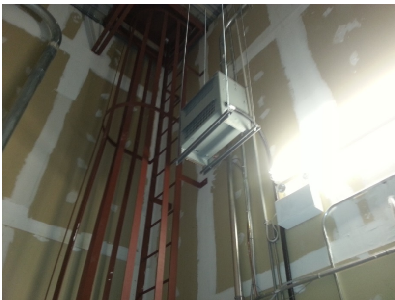
Photo 12– Dry core transformer in each unit (commercial retail units). Most are raised off the ground to save space.
