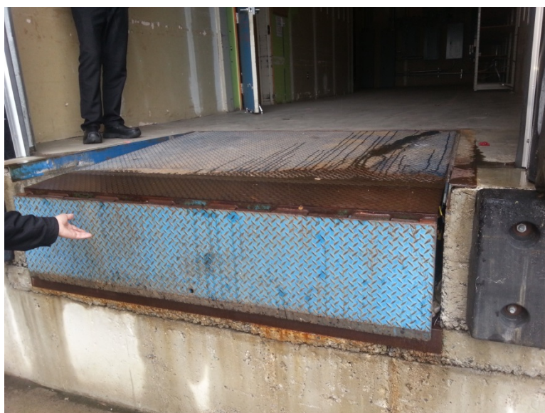
Photo 4 – Hydraulic Lift at Loading Dock (southern side of commercial retail units).
