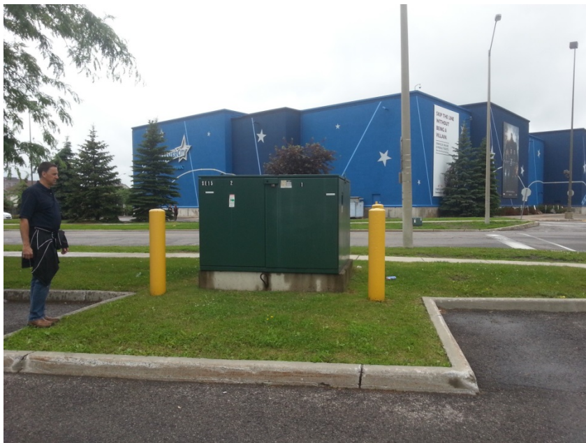
Photo 26– Pad mounted transformer.
