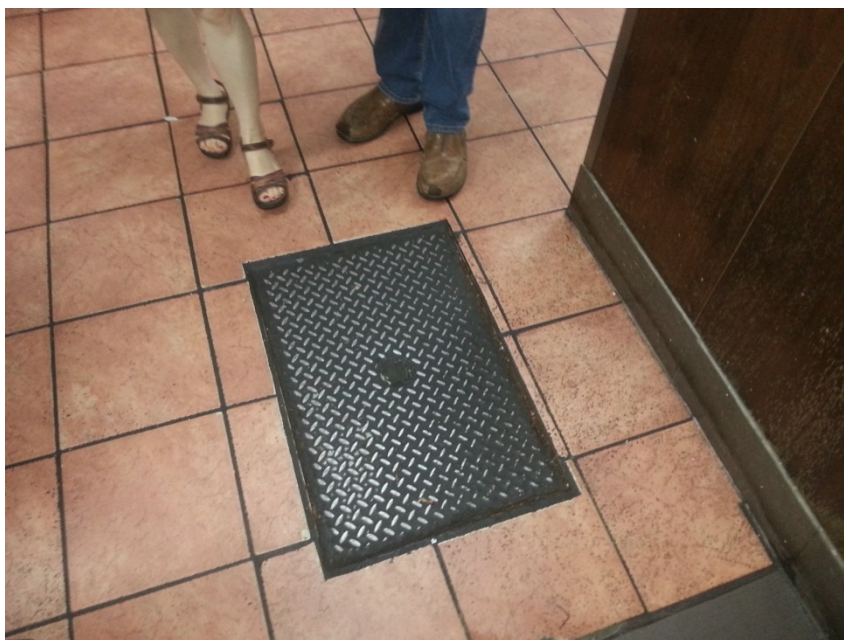
Photo 24– Second grease trap in the restaurant.
