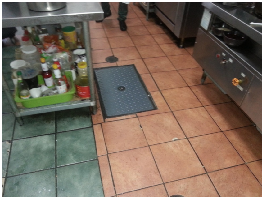
Photo 23– Grease trap in the restaurant.
