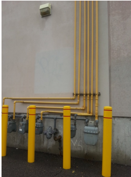
Photo 9 – Natural Gas lines running to the roof of the commercial retail units (south wall).
