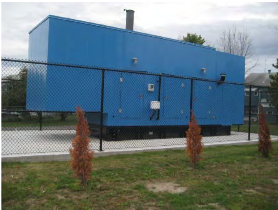
Photo 18: Standby power system with internal AST for fuel. North of new Carleton Lodge – approximately 100 m north of the Site. No staining noted on pad.
