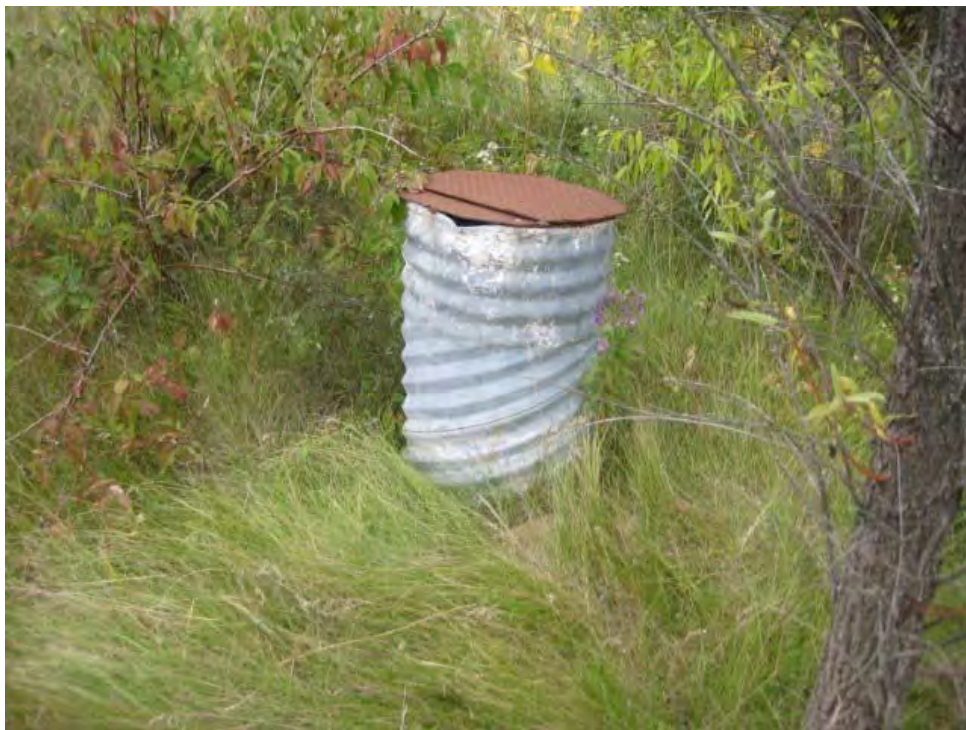
Photo 14: An abandoned water supply well on the Site of the original Carleton Lodge. The well is welded closed.
