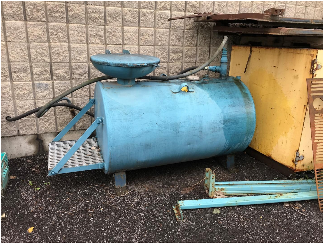
Photograph 23: Waste oil AST on the north side of the Garage Building. There was water on the right side of the tank from the rain water dripping from the sheet metal (August 2019).
