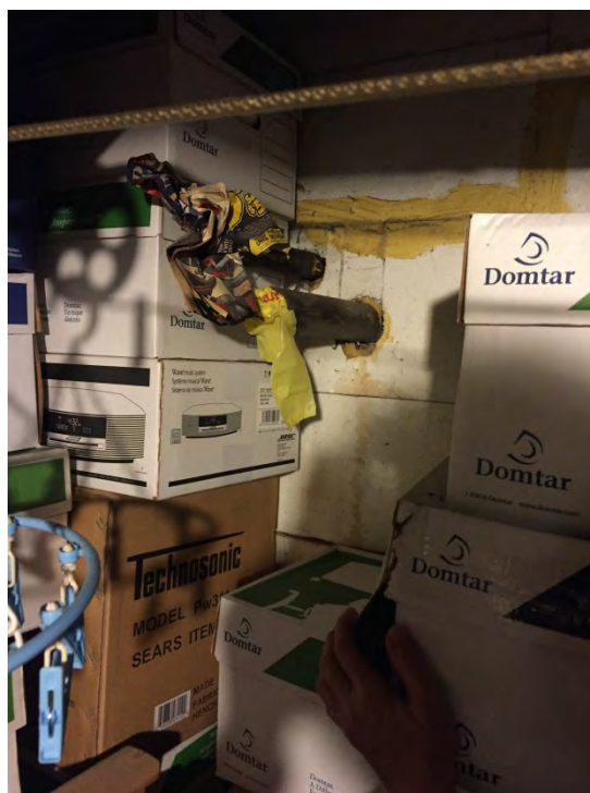
Photograph 6: Photo of the fill and vent pipes for the former fuel oil AST that have been cut off and stuffed with newspaper. This photo was taken by the Site Representative from the basement of the house.
