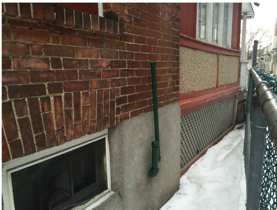
Photograph 4: View of fill and vent pipes in the basement foundation on the north side of the on-Site residential building associated with a former fuel oil ASTs.
