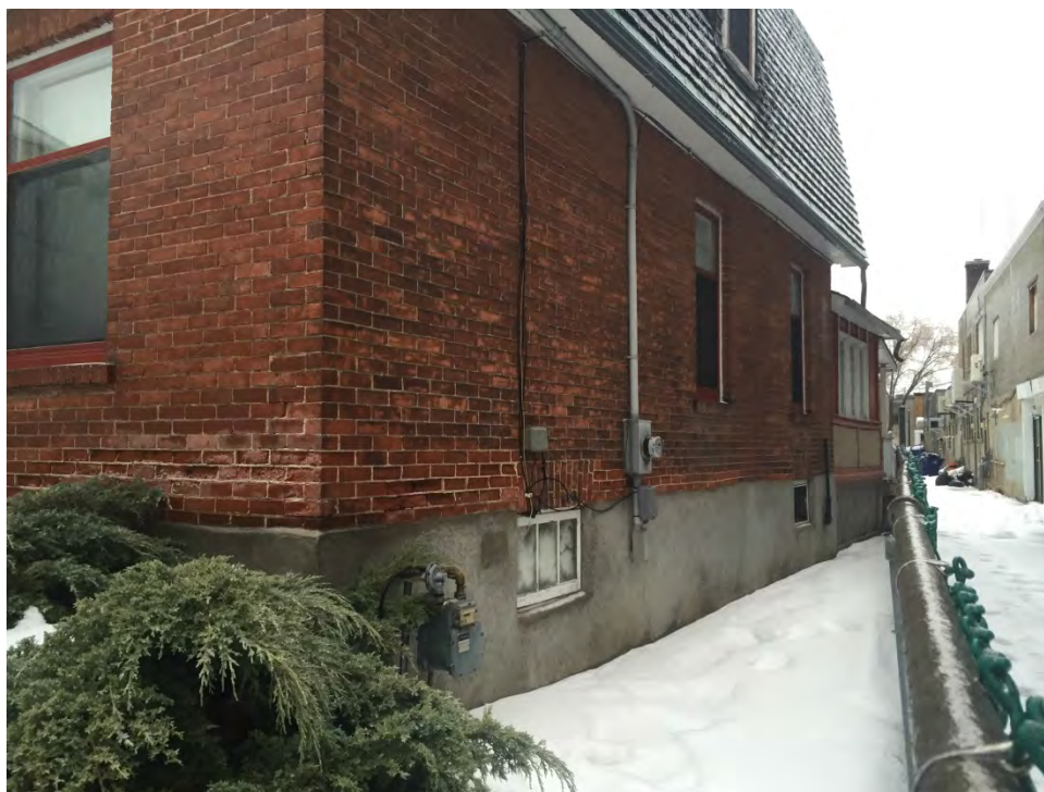
Photograph 5: Looking southwest at the natural gas meter, hydrometer and fill and vent pipes of the former fuel oil AST located along the northern exterior wall of the residential dwelling.
