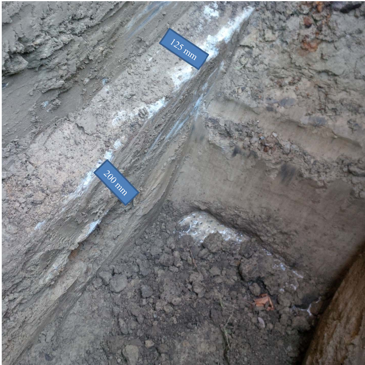
Photo B2: Strip Footing at Test Pit 2 – USF at 1.5 m below Grade – Elevation: Founding Material: Silty Sand
