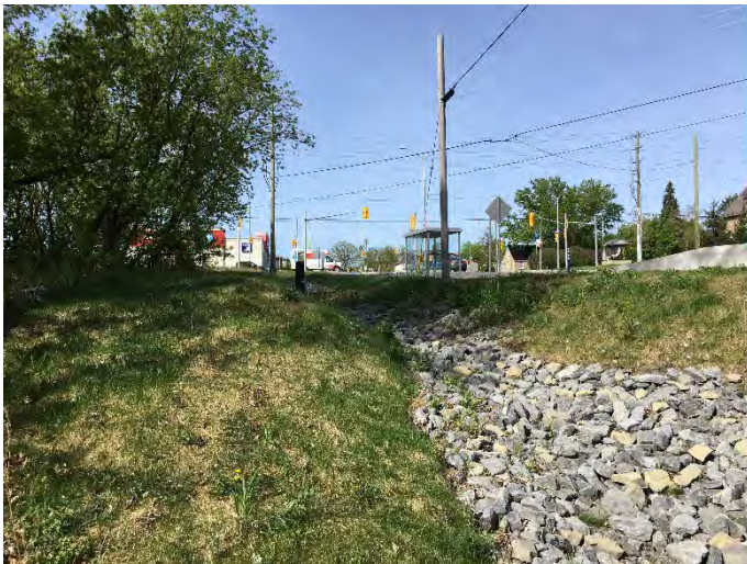
G – Drainage swale with rip rap, northern boundary of site along Klondike Road, looking southwest
