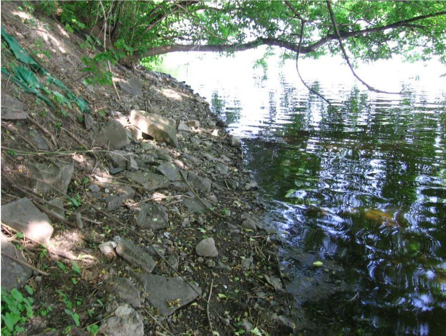
Photo 13. Shoreline showing broken concrete and unconsolidated material that has been moving downslope toward the river. While the Manitoba maples provide overhead shade, the shoreline itself lacked riparian vegetation – May 25, 2010.
