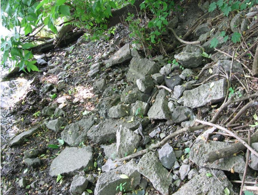
Photo 12. Shoreline showing broken concrete that has been moving downslope toward the river – May 25, 2010.
