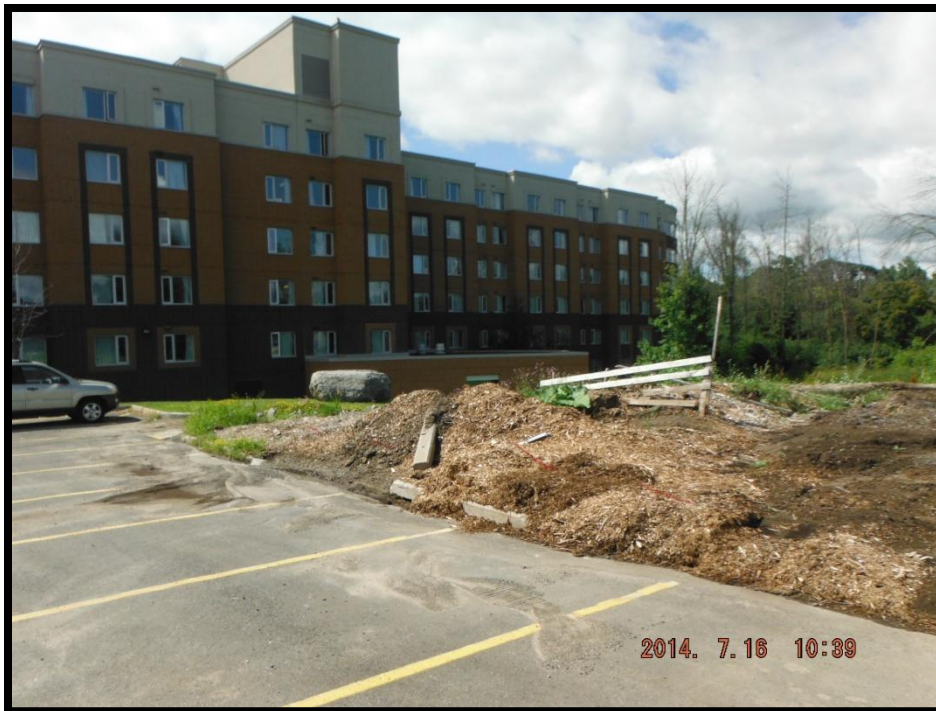
Photograph 2: View of southwest portion of the parking lot. Photograph depicts fill at apex of the escarpment, as well as, the location where surface sheet flow is diverted.
