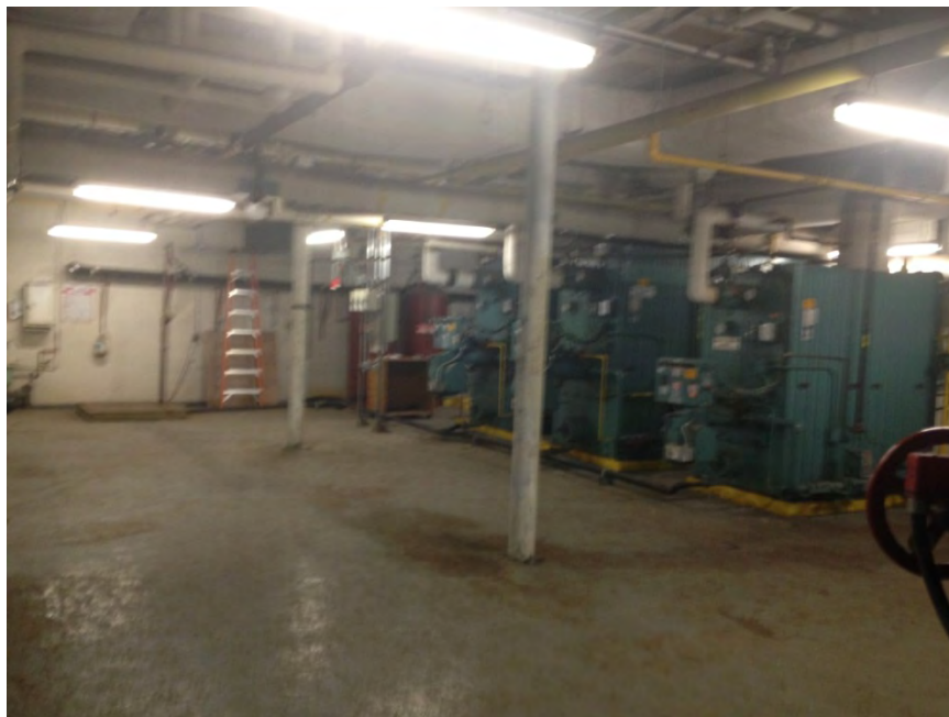
Photograph No. 3 Southern mechanical room area
