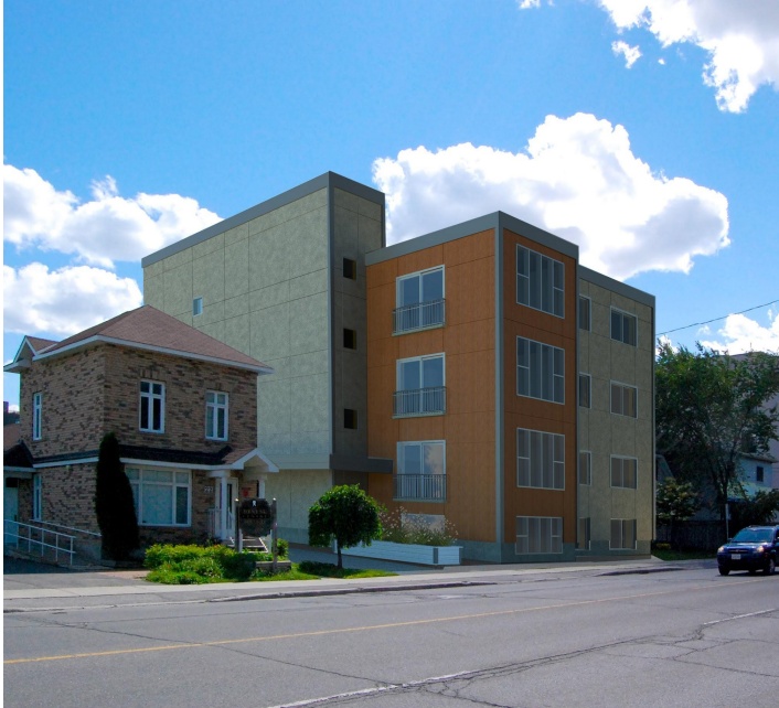
View of Site from North East
