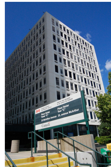
View of Adjacent Site, 25 McArthur Avenue
