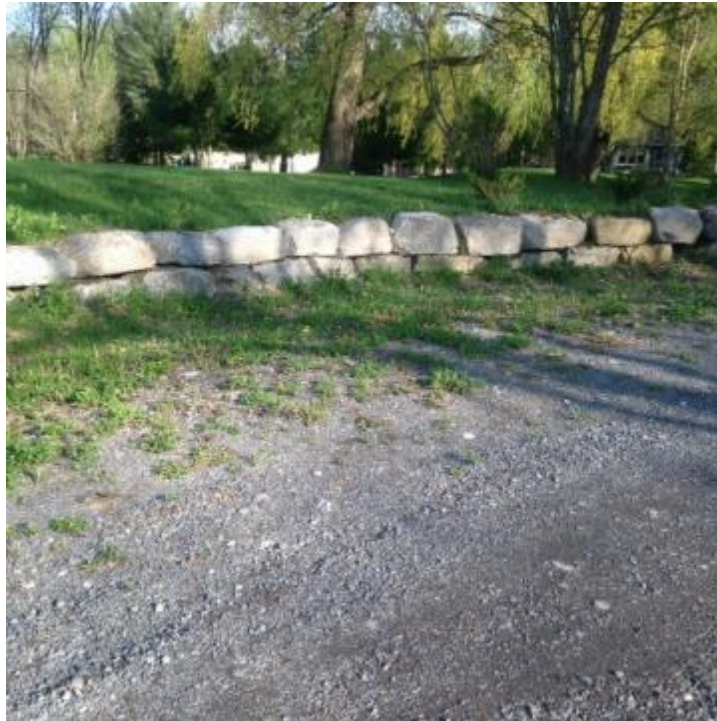
Photo No. 30 – Retaining wall at the entrance to the sanctuary.
