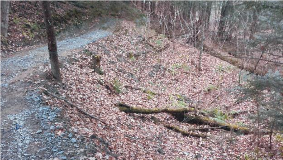
Photo No. 7 – Erosion of slope downhill of pathway. Area approximately 30 m long x 1 m to 3 m high.
