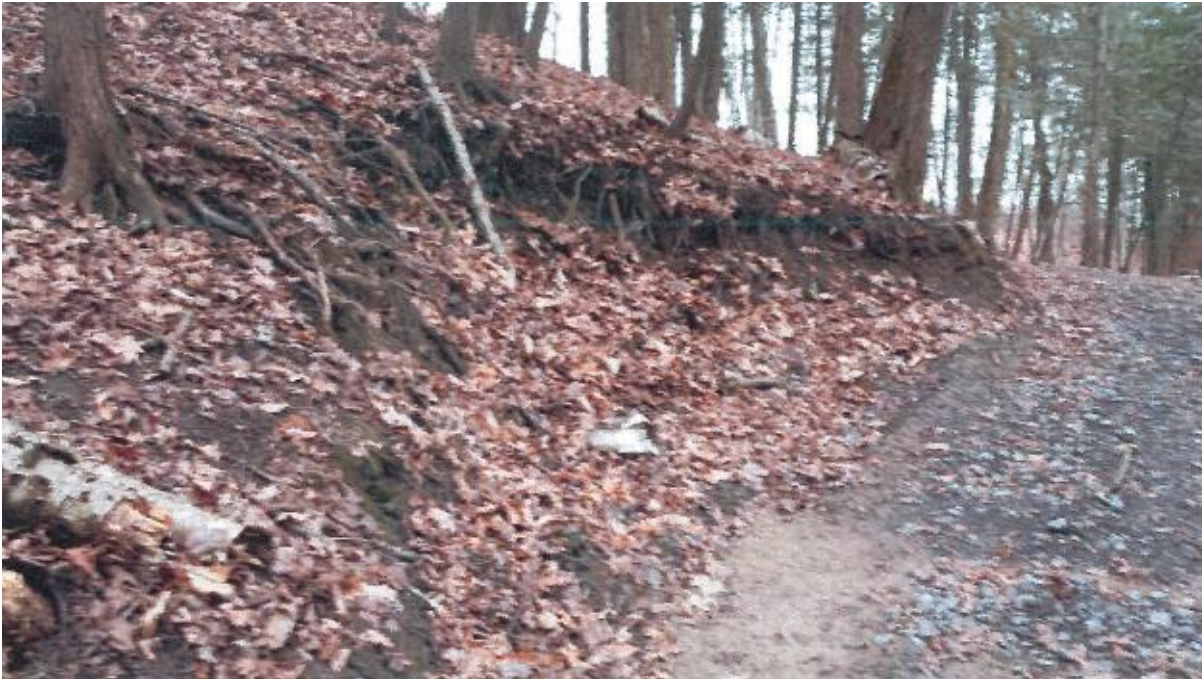
Photo No. 13 – Erosion of slope uphill of pathway. Area approximately 5 m long and 1 m to 1.5 m high.
