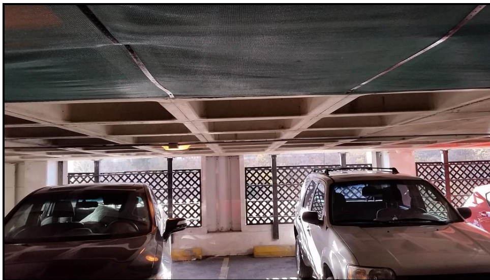
Photograph 2. View of netting in the foreground that covered portions of the ceiling
