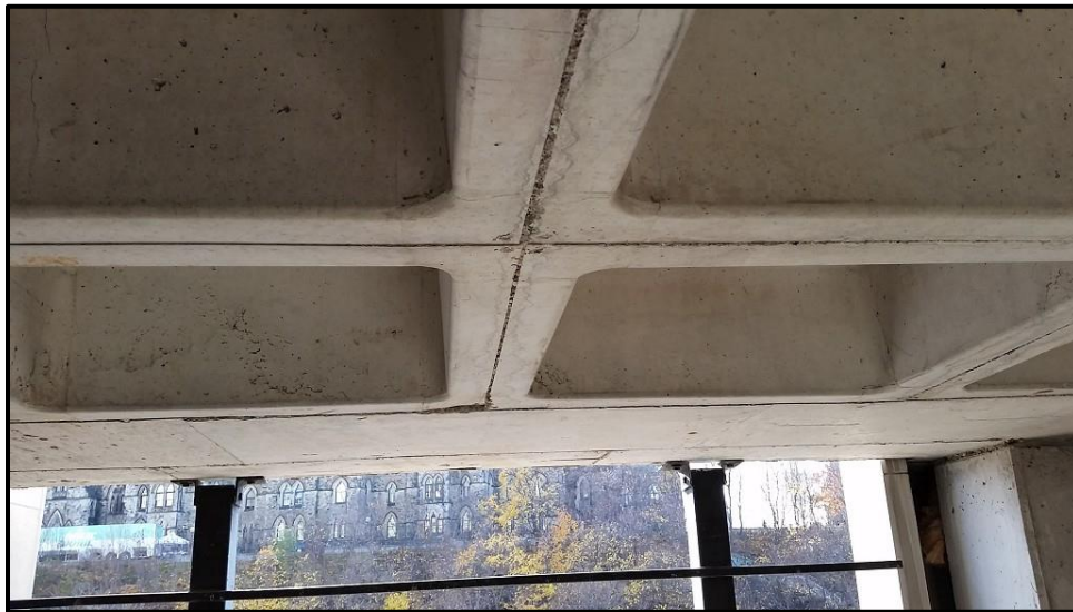
Photograph 1. View of gridded ceiling (cells 0.76 x 0.76 m with a depth of 0.3 m)
