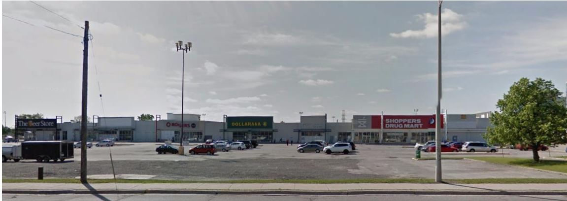
Exhibit 'B1' – Site Photo (Ogilvie Road frontage)
