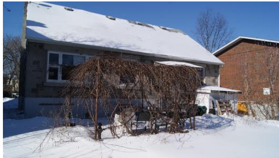
View from backyard (SE)
