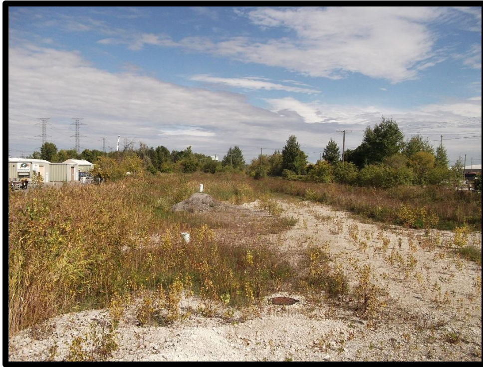
Photograph 7: Facing east from central portion of site. Note manhole in foreground and pipes over water connections.
