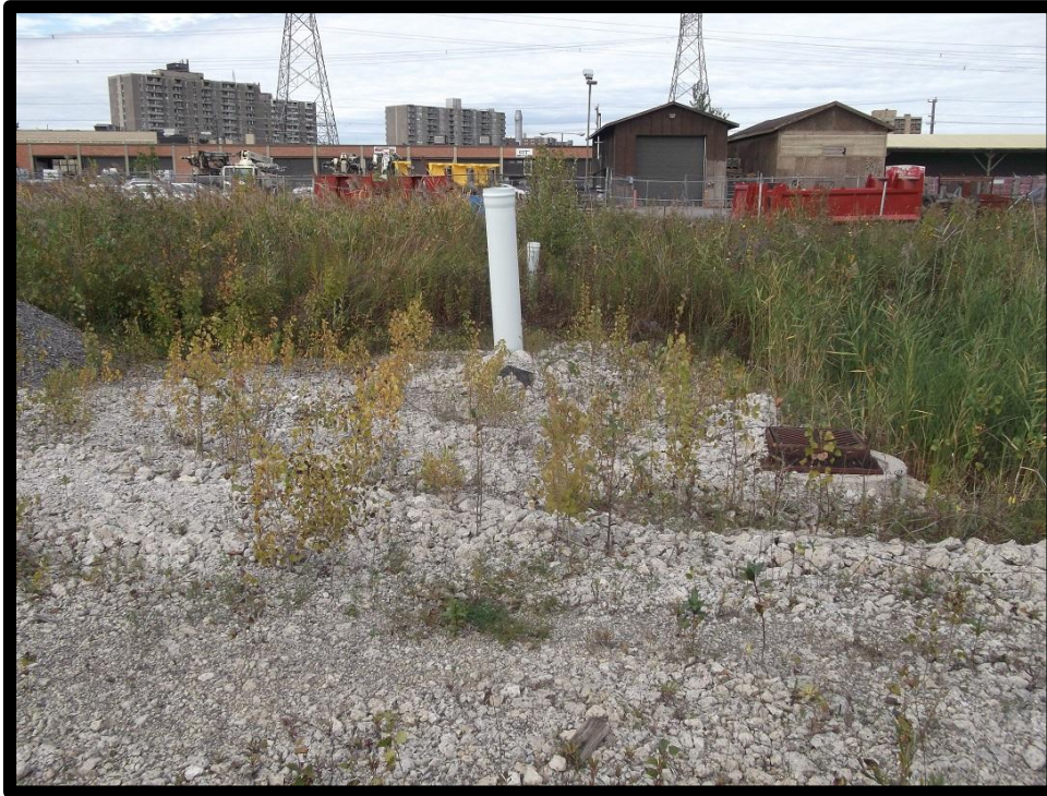
Photograph 5: Facing north from central portion of subject site, showing catch basin and pipe over water connection. Multi-unit industrial-commercial building and outbuildings (3091 Albion Road North) in background.
