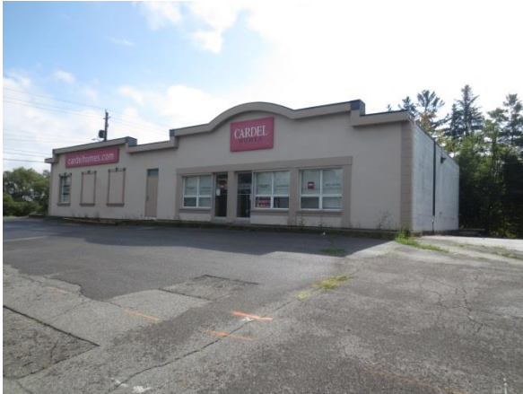
1. View of the exterior of the Phase One Property facing northeast.
