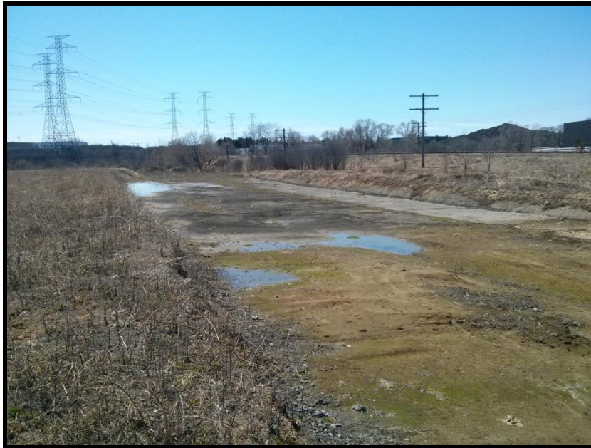
Photograph 7: View of the conveyance swale, facing southwest.
