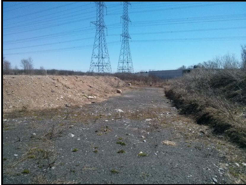
Photograph 6: View of the western edge of the raised fill area, facing south.
