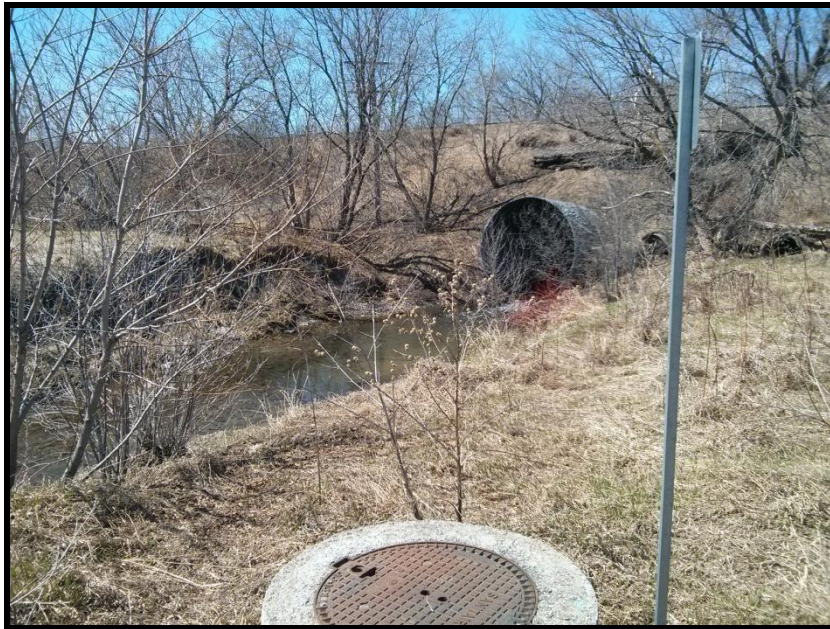
Photograph 5: View of the drainage ditch and railway embankment, facing north.
