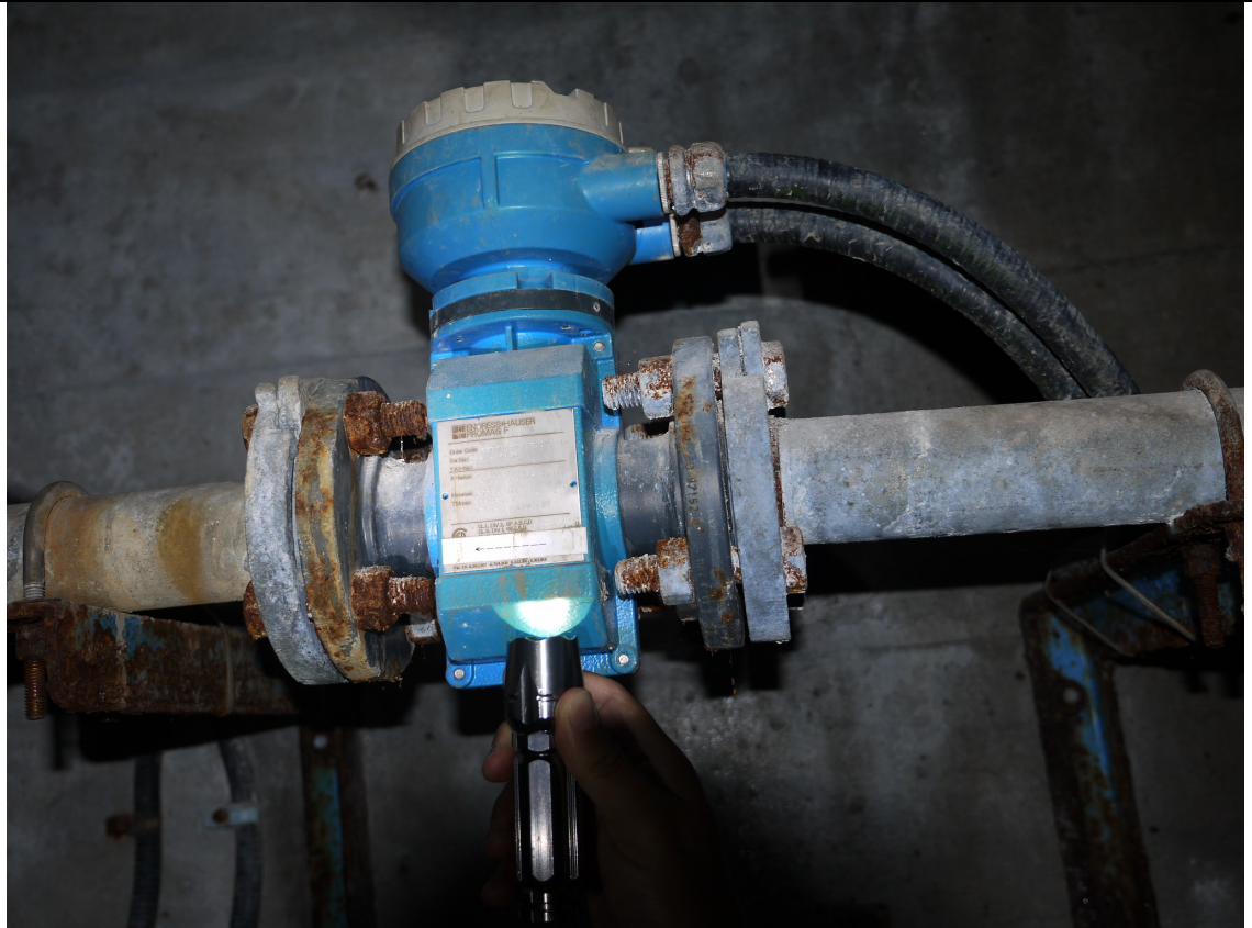
Photo 1: Flow meter: Endress + Hauser ProMag F
