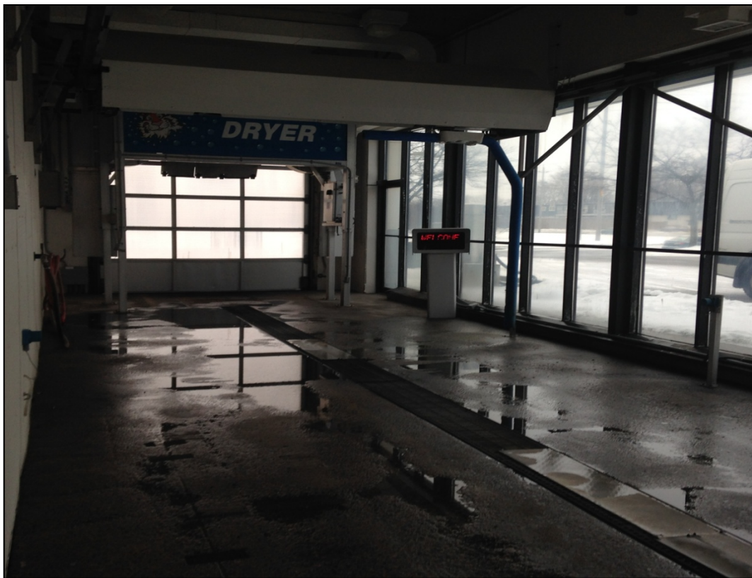
PHOTO 10: Inside the Car Wash, looking south.
