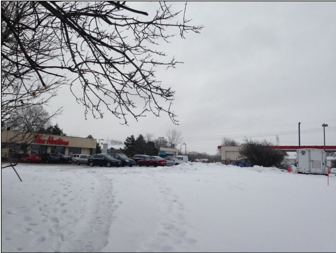
PHOTO 9: The Site, facing southeast.
