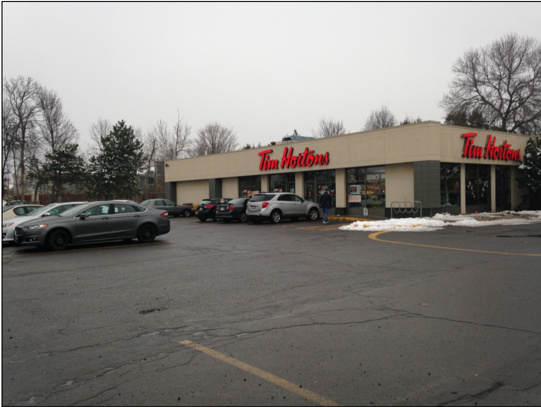
PHOTO 3: Building on-site (Tim Hortons restaurant), looking northeast.
