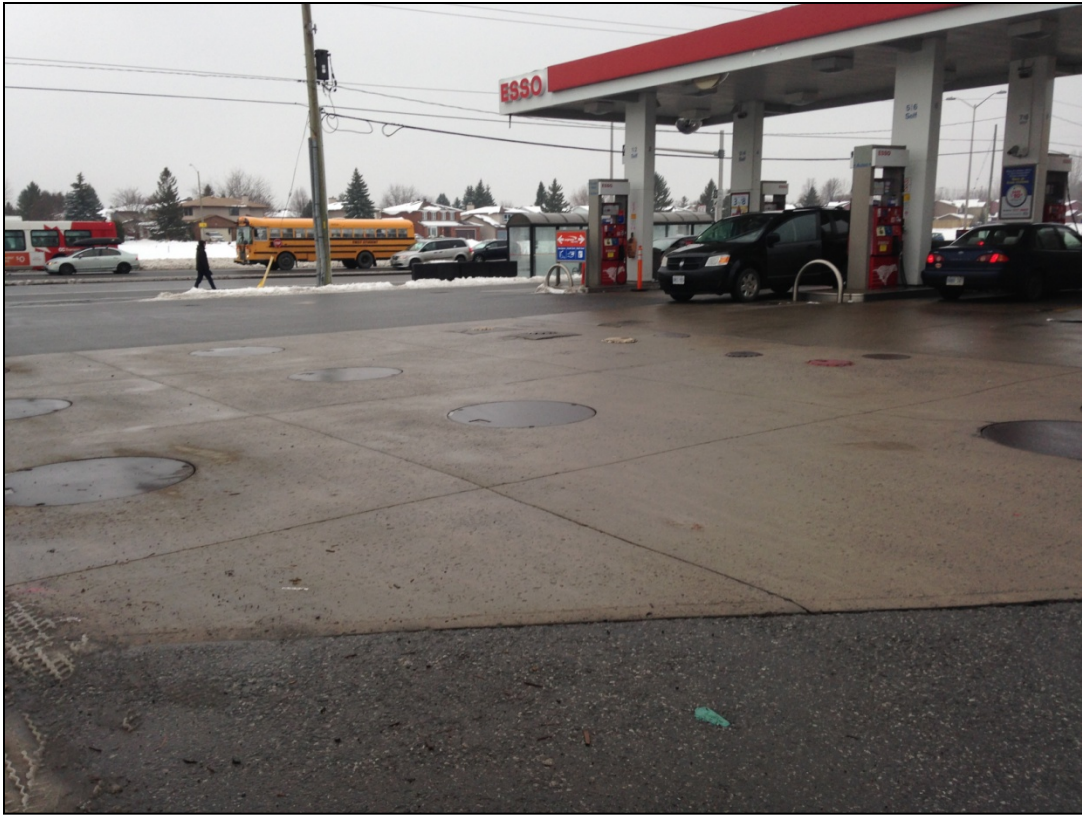
PHOTO 5: Underground tank nest area and pump islands on-site, looking west.
