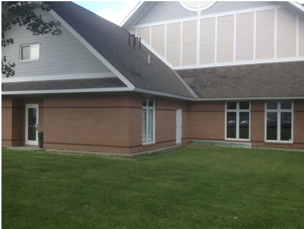
West side view of church
