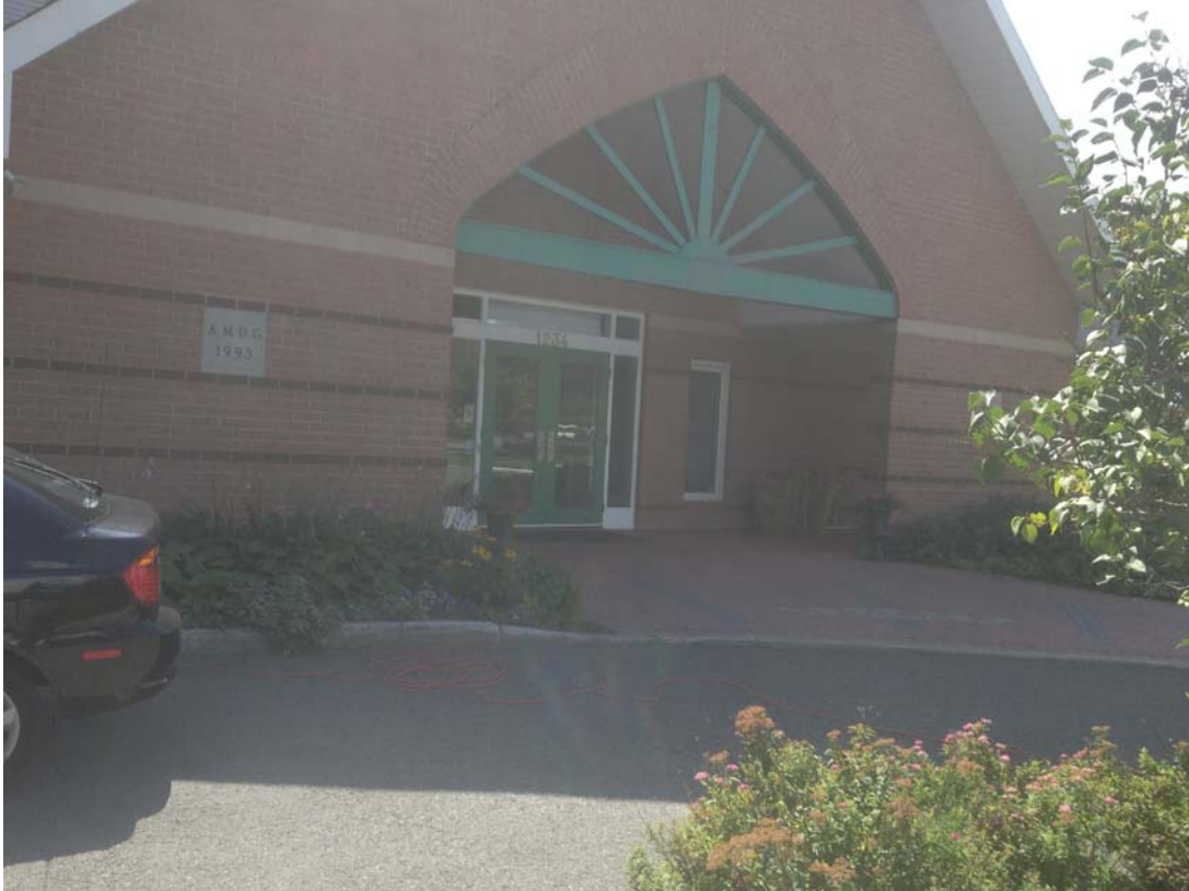
Church entrance (north side of building)
