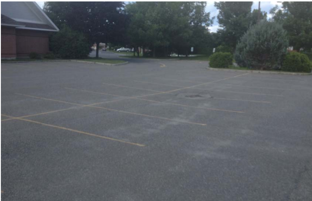
Parking lot area and entrance
