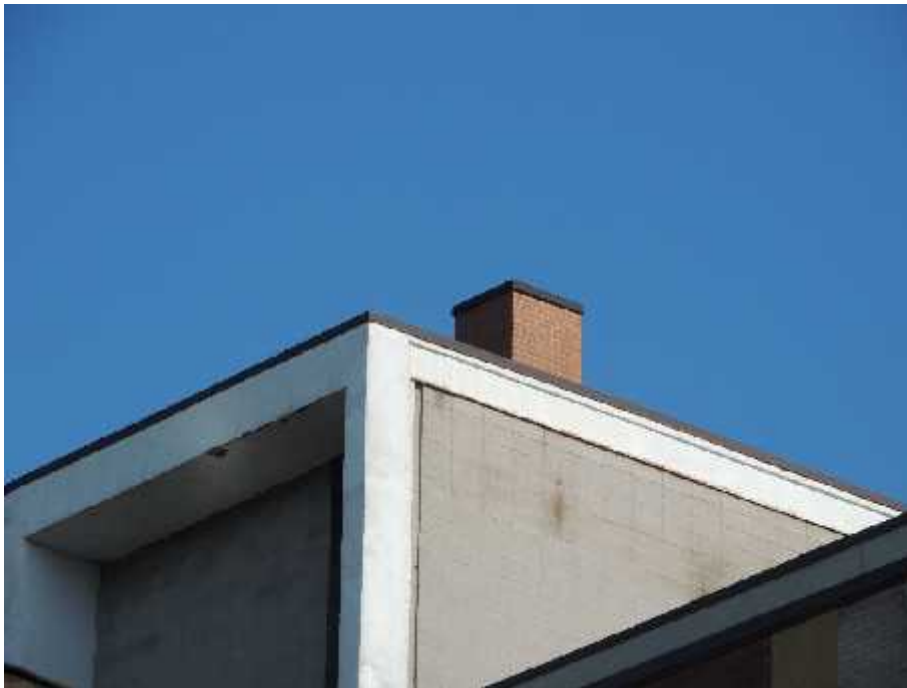
Photograph 1: Potentially uncapped chimney at 200 Bronson Avenue looking northeast.
