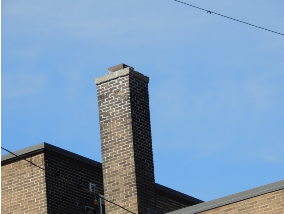
Photograph 15: Building at corner of Laurier avenue West and Bronson Avenue, chimney capped (chimney close-up).
