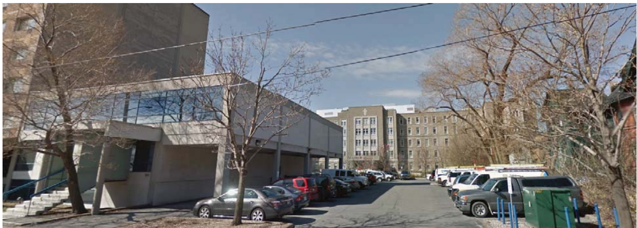
FIGURE 2: EXISTING TWO-STORY OFFICE BUILDING ON THE SUBJECT PROPERTY
