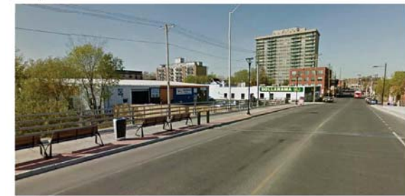
6 VIEW LOOKING WEST ON SOMERSET FROM BRIDGE NTS
